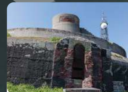
Brickwork construction (underground part of the central turret)
